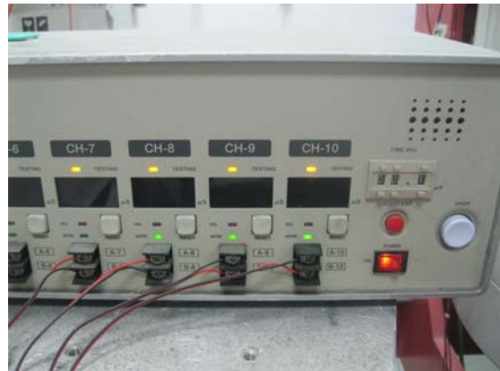
monitor during the test
