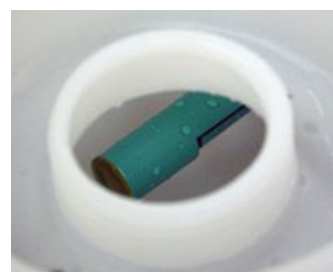
Figure 6: Chiller Low Level Switch
